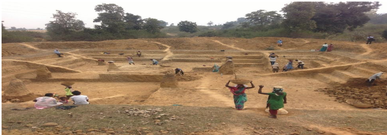
Work – Pond Constructin, District – Simdega
