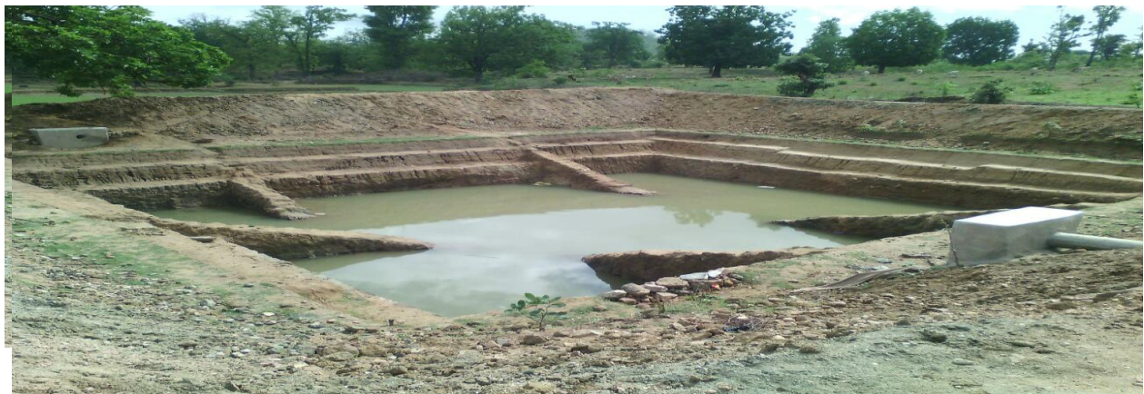
Work – Pond Constructin, District – Simdega
