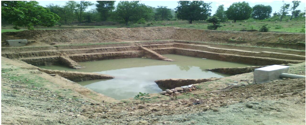
Work – Pond Constructin, District – Simdega
