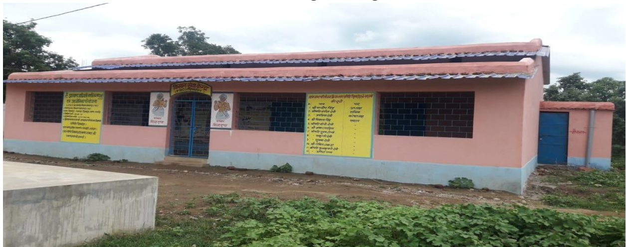
Work – FCC, Village – Barwadih, Barwadih, Latehar
