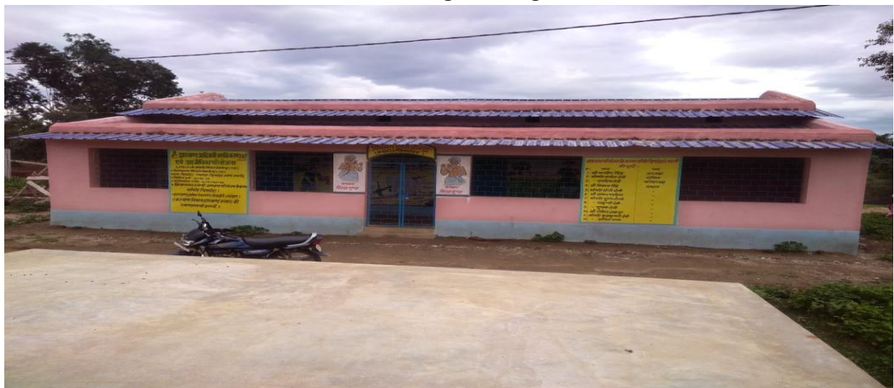
Work – FCC, Village – Barwadih, Barwadih, Latehar
