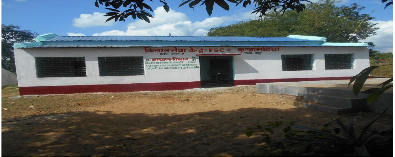
Work – FSC Centre, Village – Kundamatia, Amrapara, Pakur
