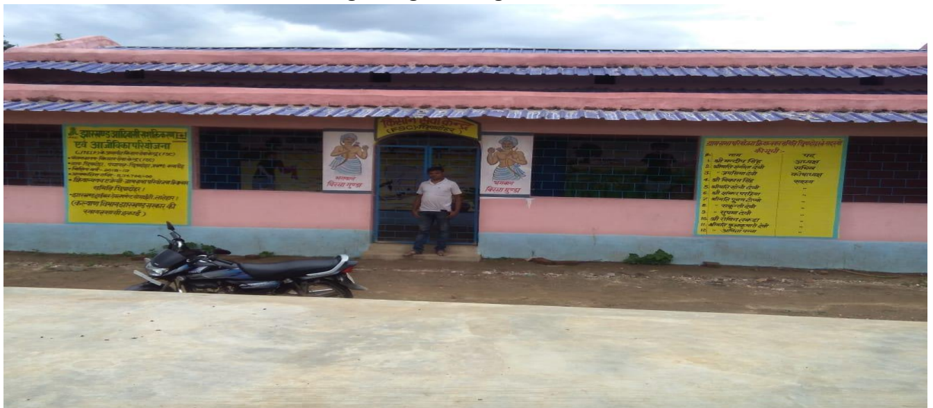
Work – FCC, Village – Barwadih, Barwadih, Latehar
