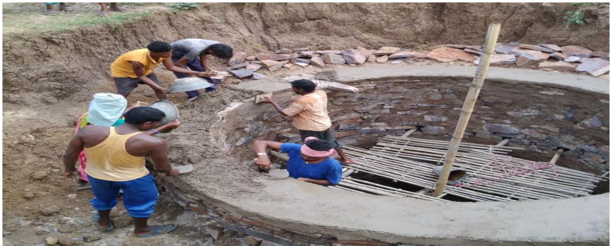
Work – Well Constructin, District – Simdega
